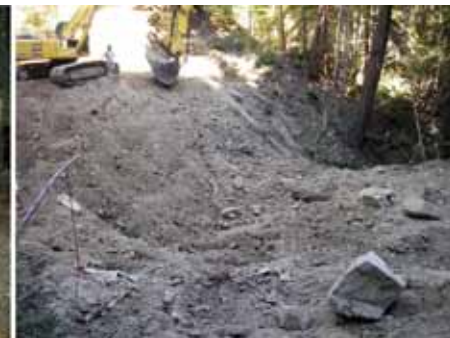
Log stringer culverts removed from Lack's Creek drainage.
